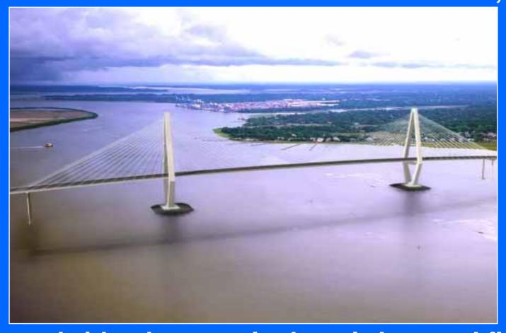
The new bridge has steel edge girders and floor beams. The total bridge length is 13,200 feet (2.5 miles) end to end.
